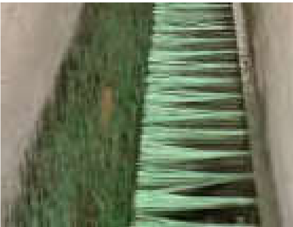
Cross section of a brush elver pass
